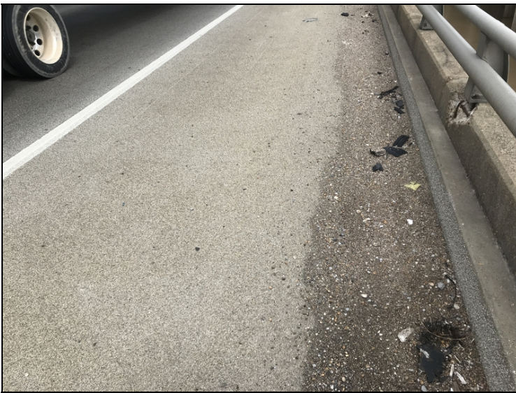
Typical debris in gutters
